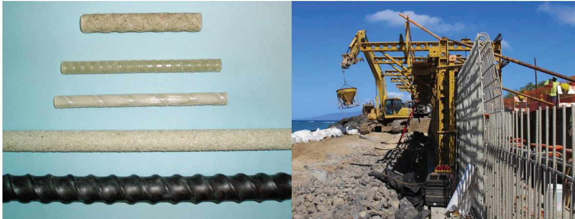
Figure 9: GFRP bars Used in Seawall in Hawaii, US (ACI 440.1R, 2015)
